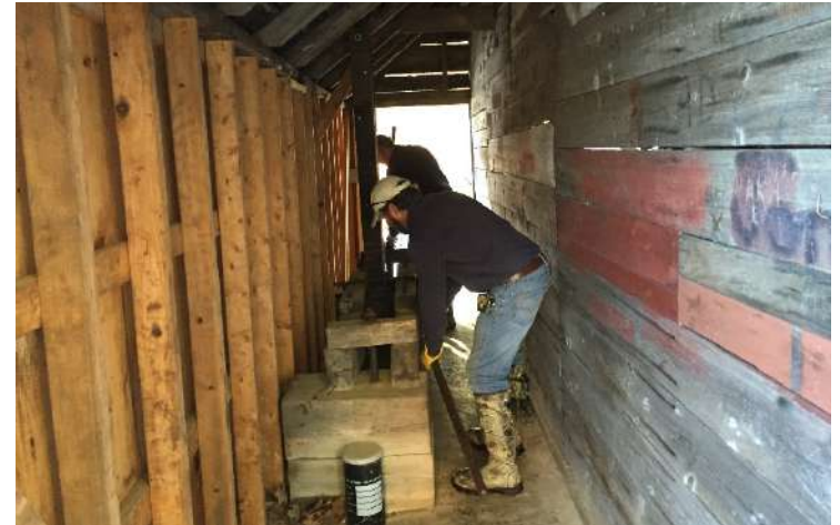
Adjusting the dam gate
