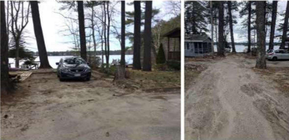
The timber frame lip overlooking the right of way to the lake in spring 2020 (left) and stormwater runoff and sediment transport evident in Spring 2019 (right).
