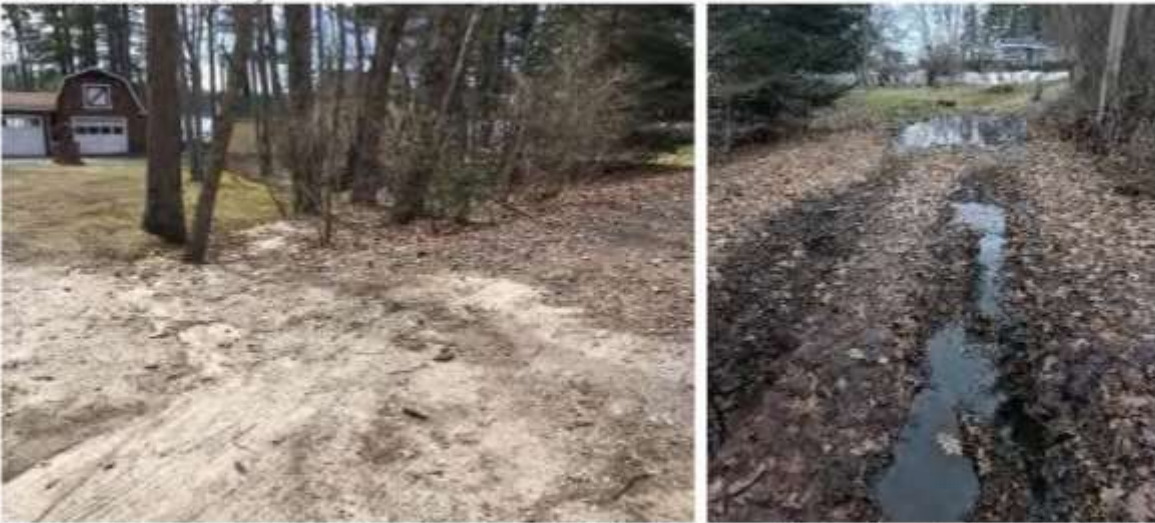
Sediment transport towards lake in spring 2020 (left) and ponding and rutting on the Watchic Road 3/Hartford Lane in spring 2019 (right).
