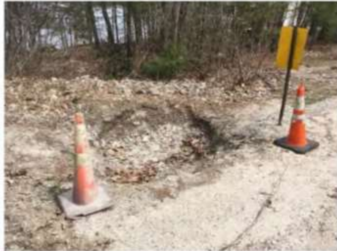
Sloped road approaching site (left), eroded hole at clogged culvert outlet (right).
