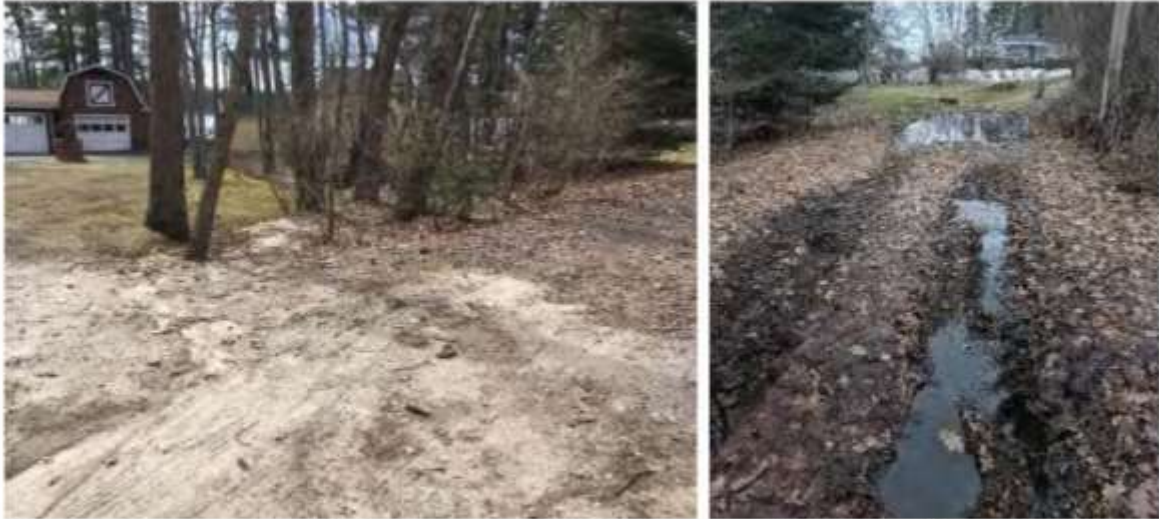
Sediment transport towards lake in spring 2020 (left) and ponding and rutting on the Watchic Road 3/Hartford Lane in spring 2019 (right).
