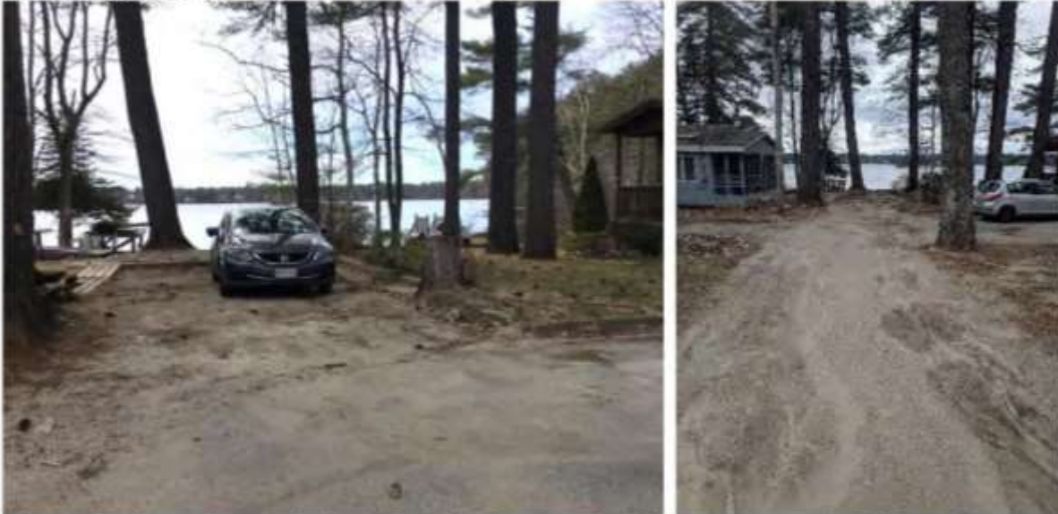
The timber frame lip overlooking the right of way to the lake in spring 2020 (left) and stormwater runoff and sediment transport evident in Spring 2019 (right).
