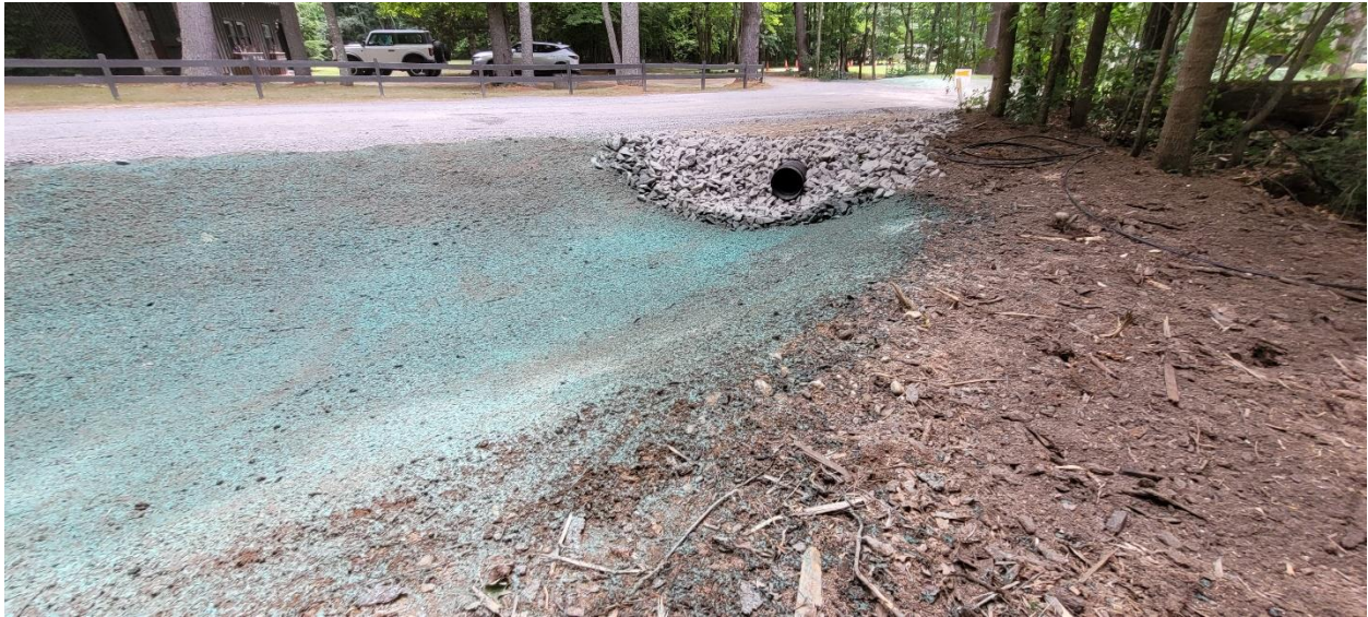
Watchic Road 3 Culvert and Retention Pond
