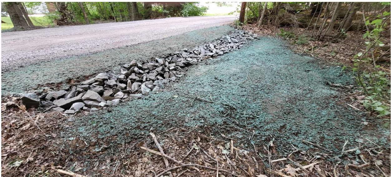
Watchic Road 3 Rock Sandwich Allowing Runoff Under the Road
