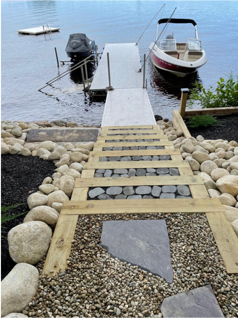
Watchic Crossroad. Permeable grout on steps and river rock on top step.
